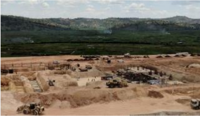
Large Area Grading
