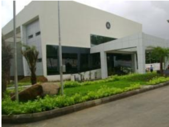
RBI Data Center, India
